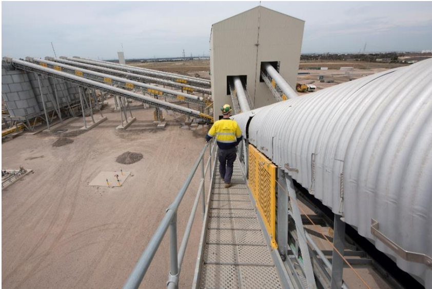
Plant upgrade at Deer Park Quarry, Vic
