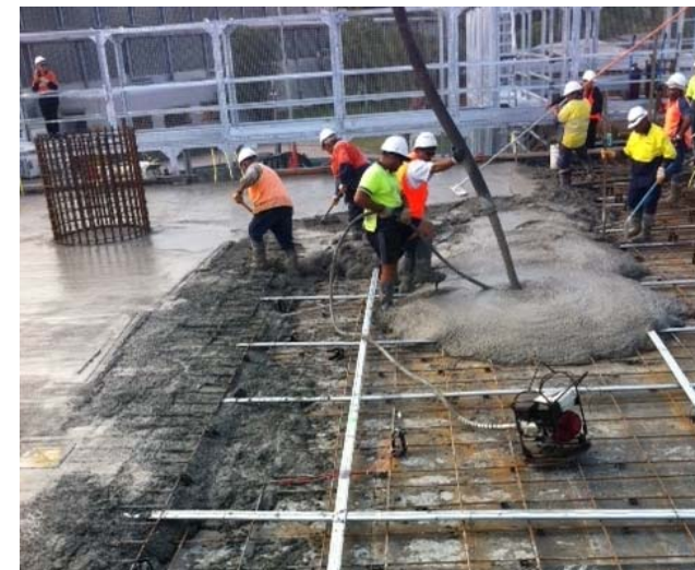
Field trials of ENVISIA ™ concrete for the Barangaroo Project
