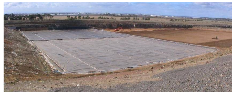
Deer Park landfill – New composite lined cell
