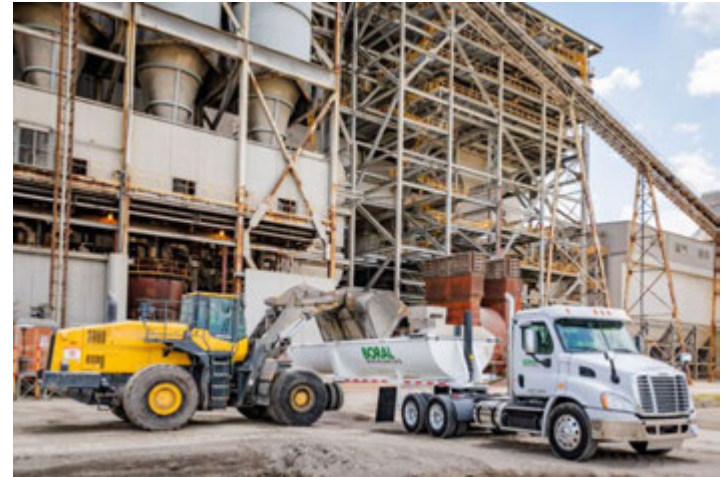
Fly Ash facility in Austin, TX
