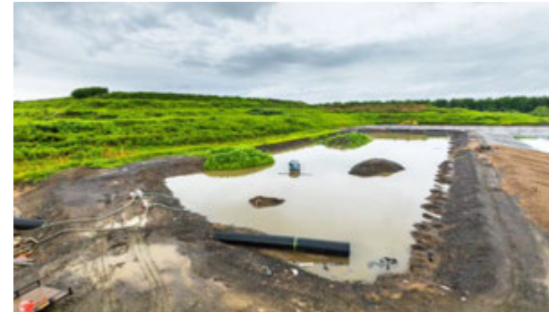
Fly ash pond at operational facility
