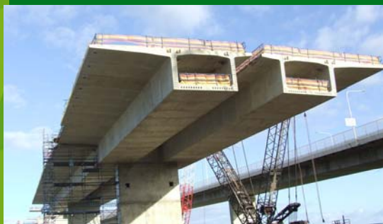
Construction of Gateway Bridge, Brisbane
