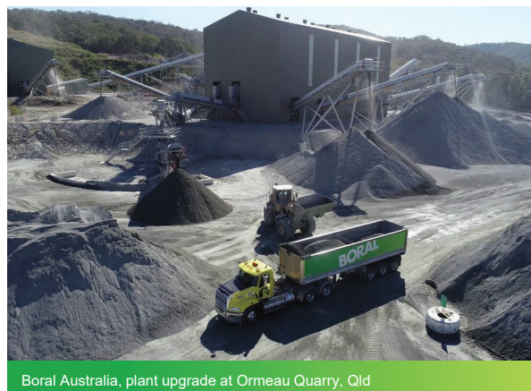
Boral Australia, plant upgrade at Ormeau Quarry, Qld
