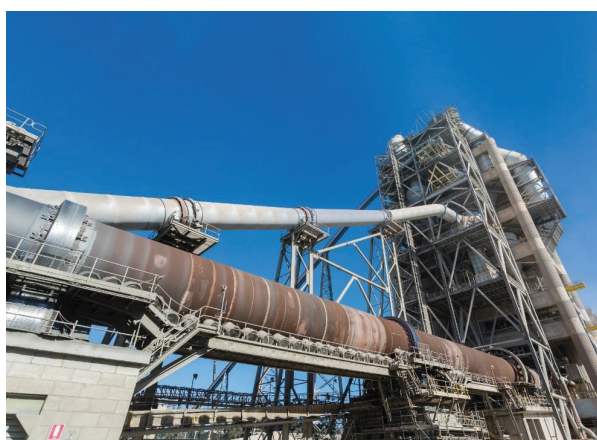
Boral Australia, Berrima Cement Works, NSW
