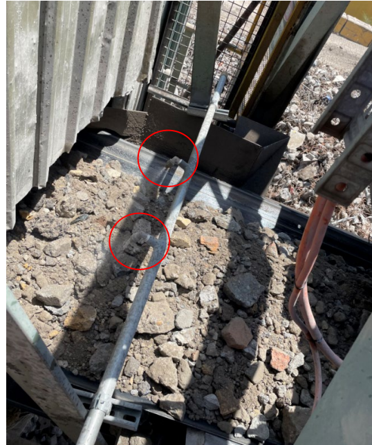
Figure 5 – Additional fixed water sprays on fixed plant
