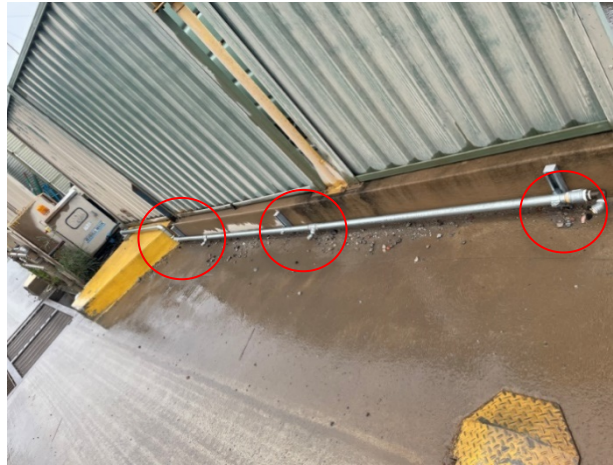
Figure 7 – Example of additional wet suppression infrastructure installed
