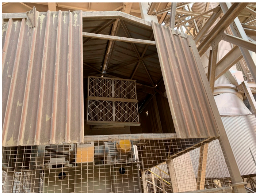
Photograph 3.1: FA38 with part of the side cover removed
