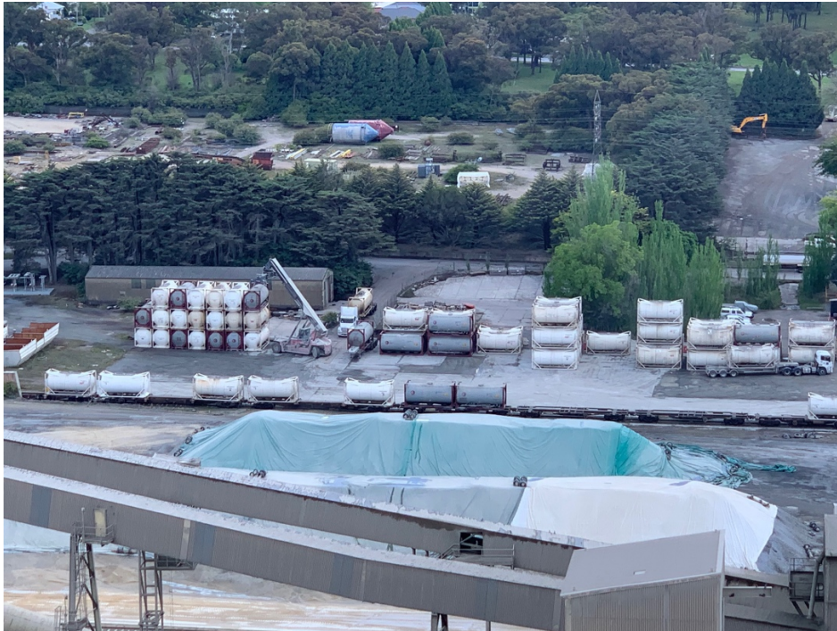
Figure 3.10 The isotainer train loading operations site viewed from the tower
