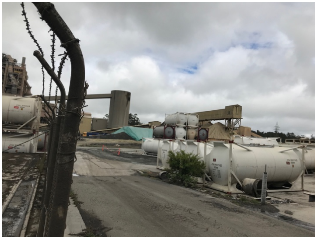
Figure 3.10 View A :- Looking down the truck loading road and at the western stack
