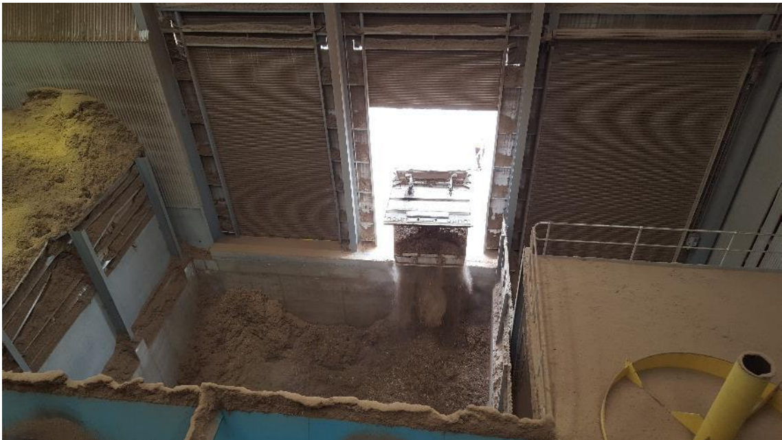
Plate 3 – Truck Vibrating to Discharge NSF into Reveal Bunker
