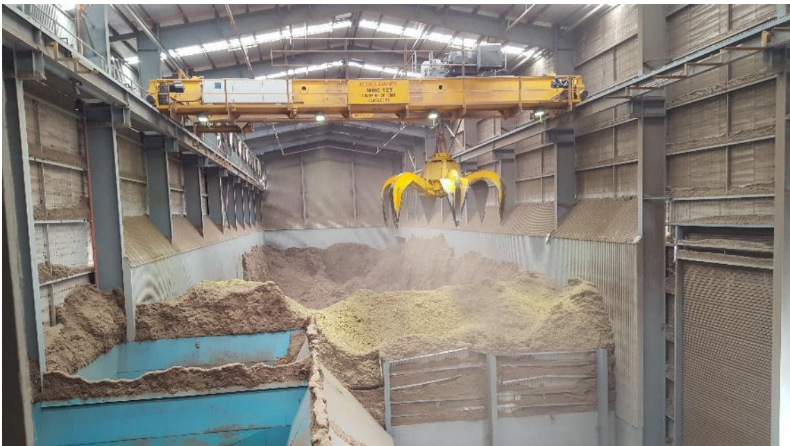
Plate 5 - Material Grab used to load conveyor system
