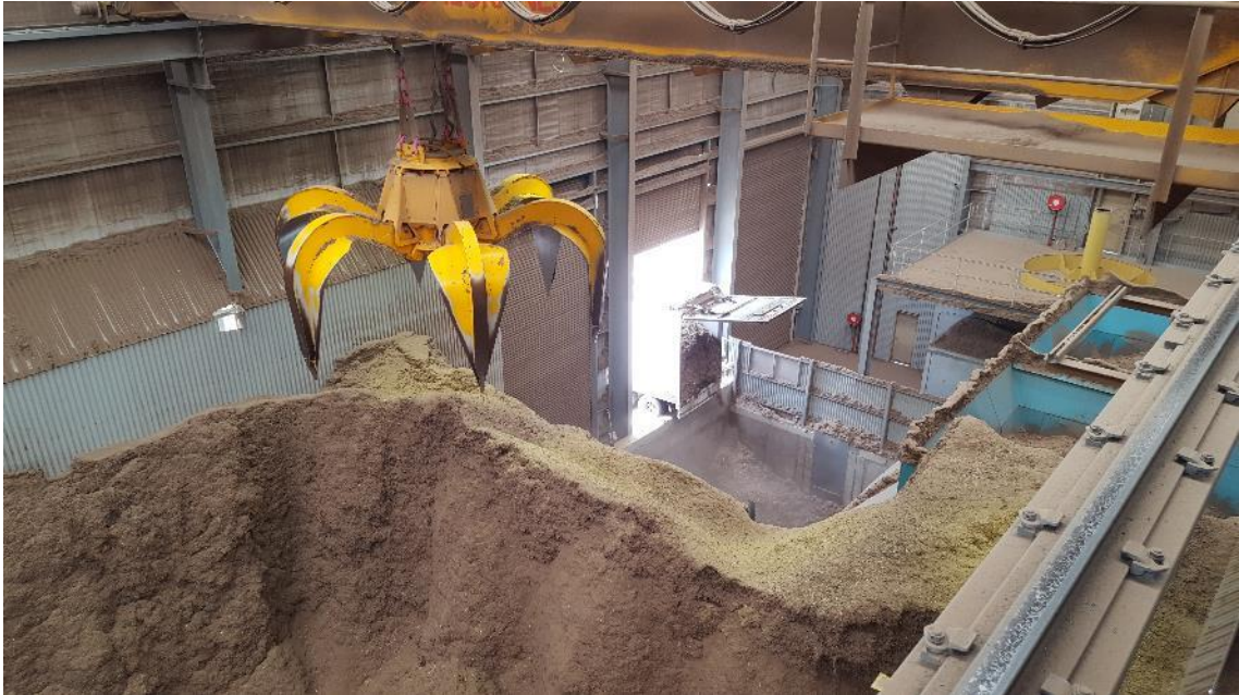
Plate 4 – Material Grab used to load conveyor system
