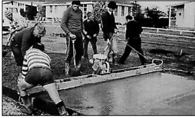
**Figure 7:** Typical surface vibrator
