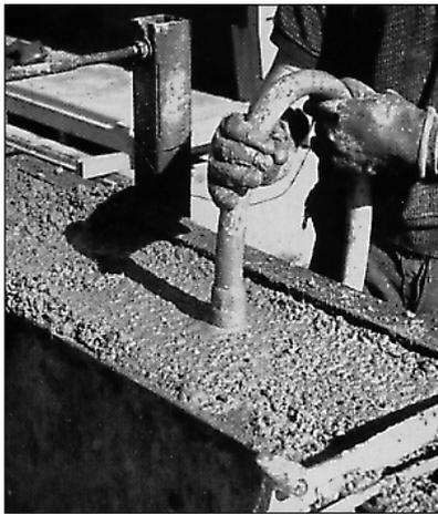
**Figure 3:** Use of an immersion vibrator
